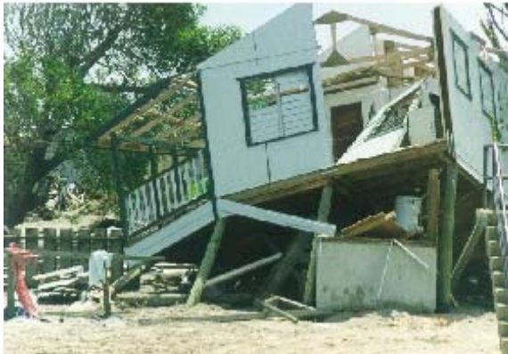
Destruction caused by Hurricane Iris on Placencia Peninsula
